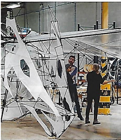
Working on details of the flying structure which required modified framing and sail materials, 2019.
