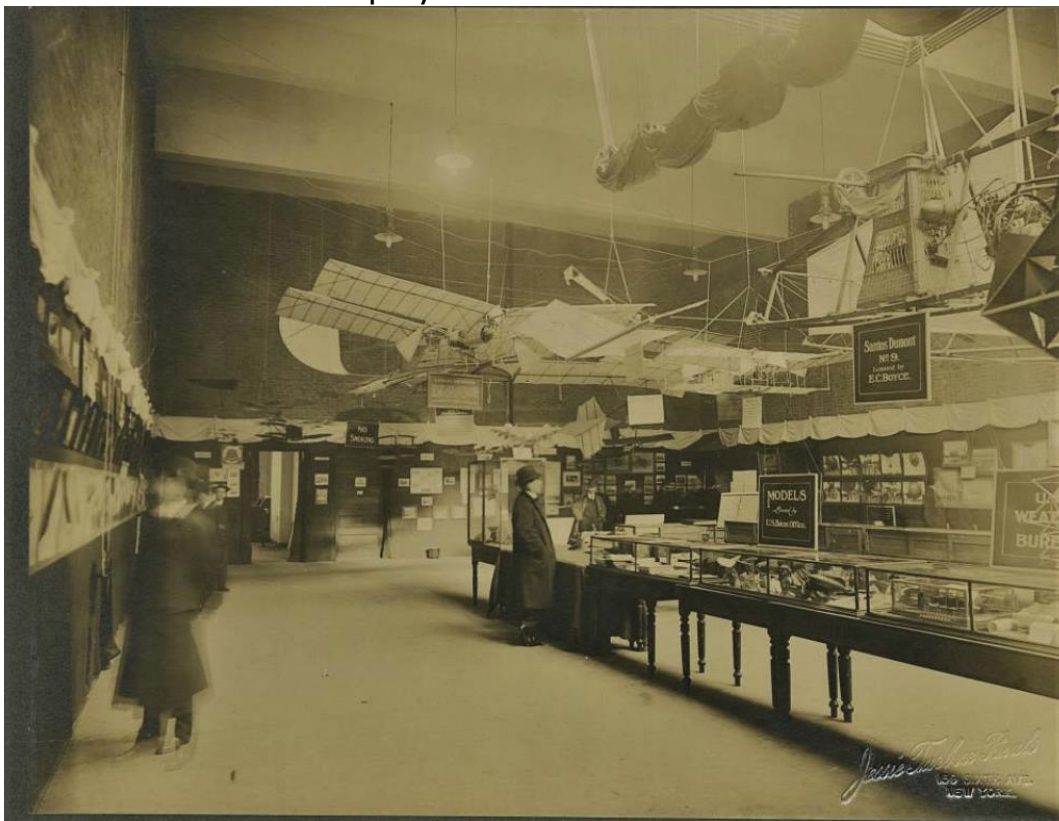
View No. 5: Looking north from center of west wall Notes: Models loaned by the U.S. Patent Office are visible in the foreground; hanging over the cases are (front to back) the Santos-Dumont (Alberto) No. 9 "La Baladeuse" airship, Hargrave (Australia) 1888 Compressed-Air Ornithopter and Herring 1902 Gasoline Biplane Model, and the 1897 steam-powered Langley Aerodrome Number
